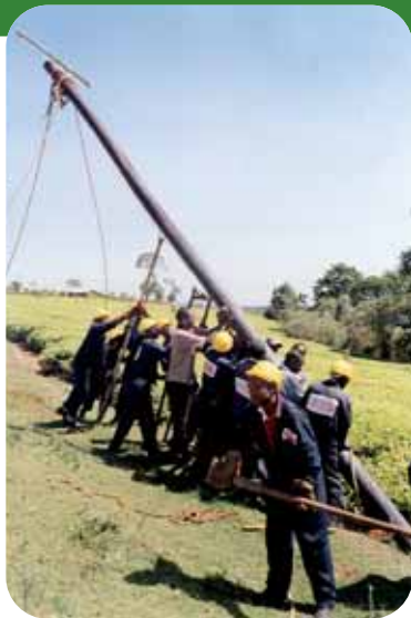
Rural electrification works
